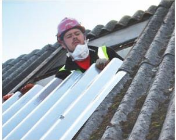
Locating replacement sheet
