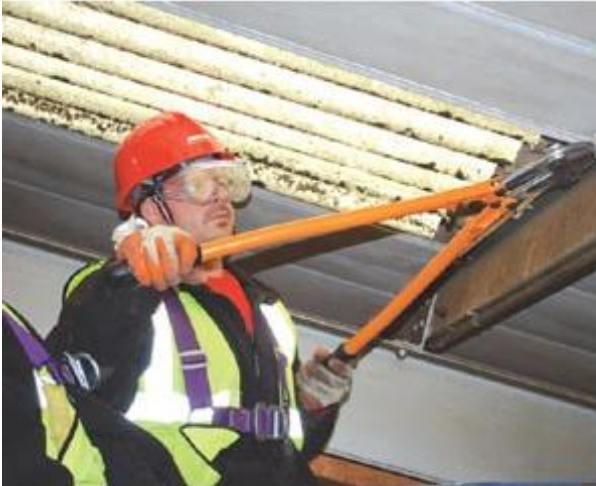
Removing hook bolts from existing sheet
