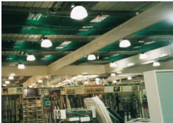
Safety netting used to provide protection for roof lights during minor roof works
