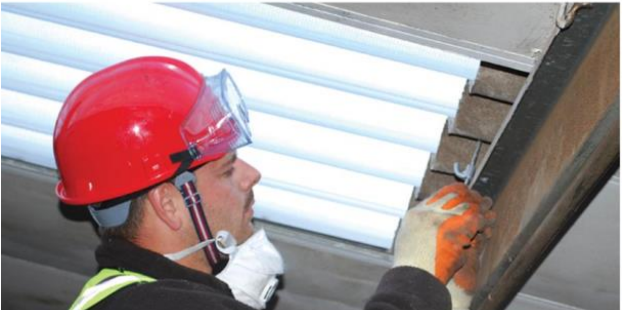
Securing fixings to newly installed sheet
