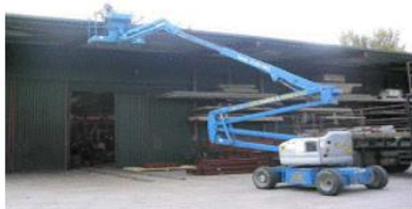
Using a MEWP to clean a gutter
