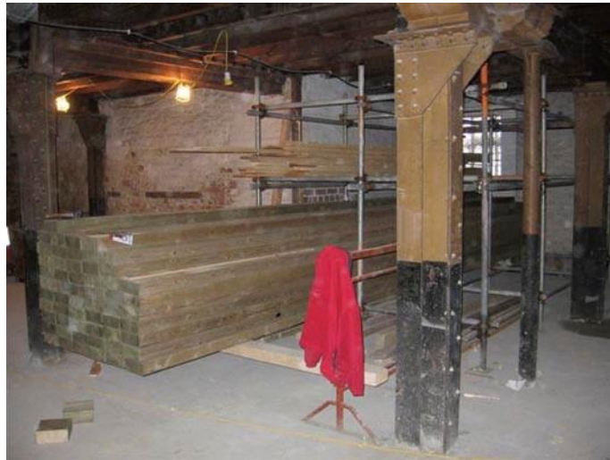
Figure 5 A designated timber storage area
