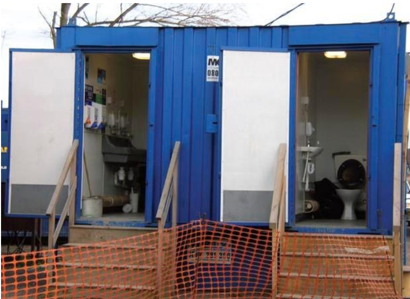
Figure 2 A self-contained water-flushing toilet block with built-in tank people to wash their forearms
