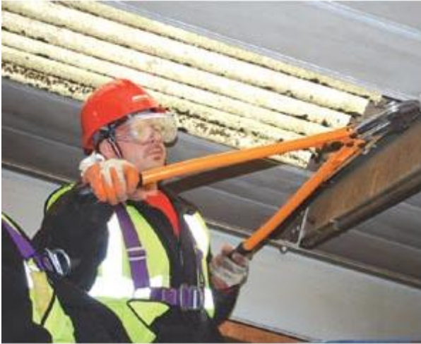
Removing hook bolts from existing sheet
