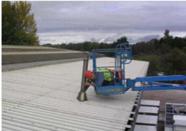
Using a MEWP to inspect a vent
