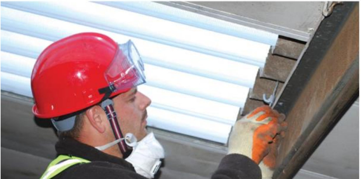
Securing fixings to newly installed sheet
