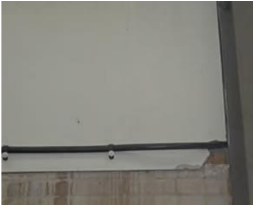
AIB soffit under roof
