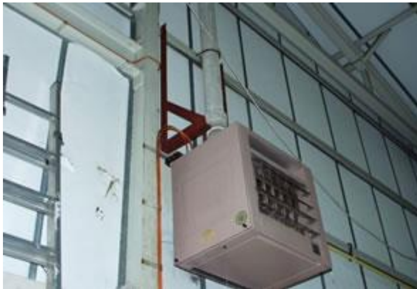
Asbestos cement flue from ventilation unit
