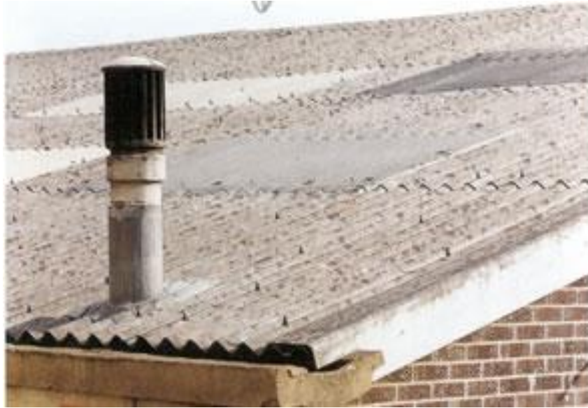
Asbestos cement roof panelling
