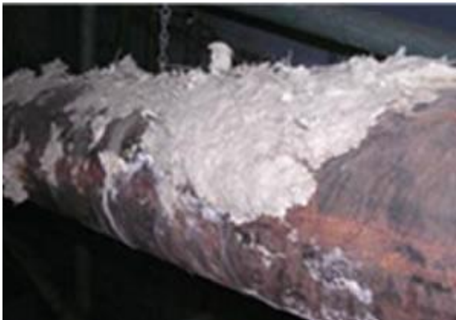
Asbestos lagging on hot water pipes
