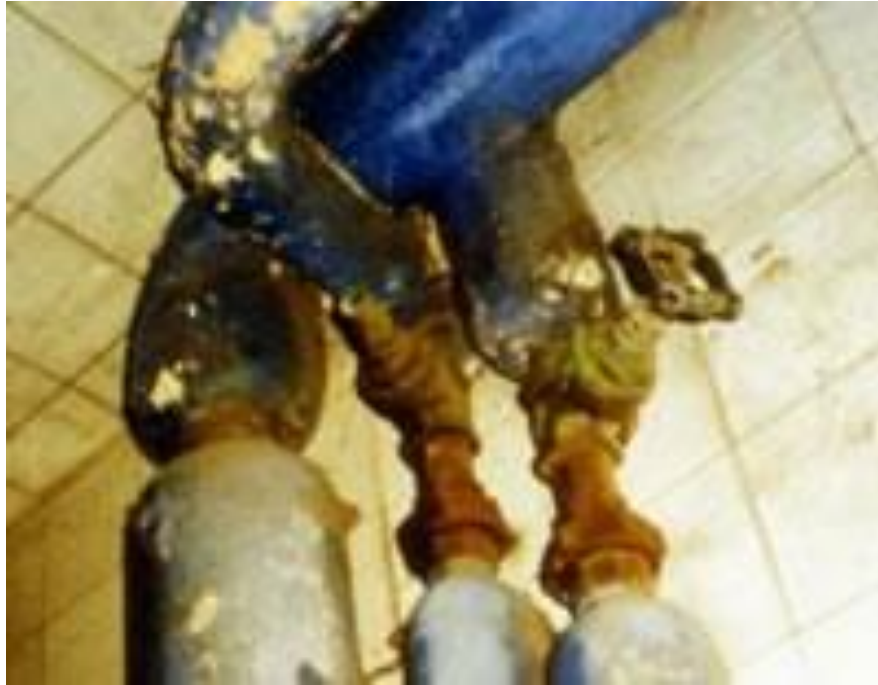
Asbestos lagging on hot water pipes
