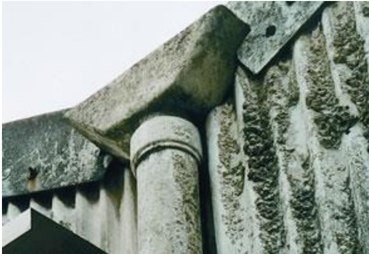
Asbestos cement downpipe, hopper and profile sheet
