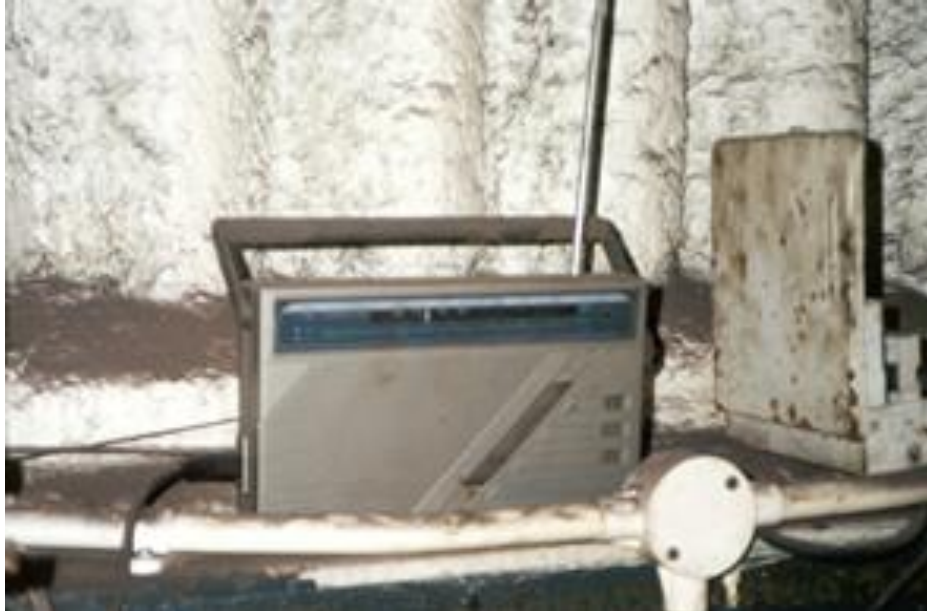
Spray Coated Panelling
