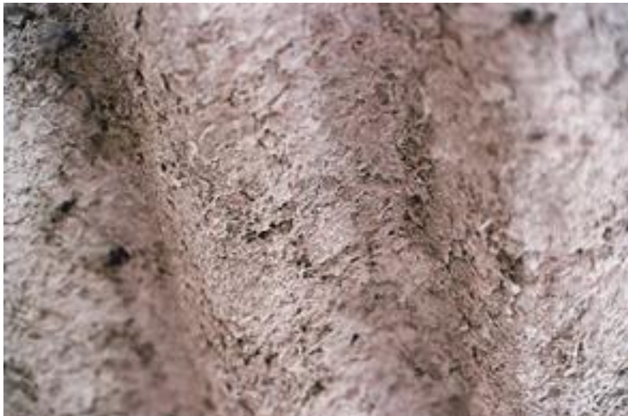
Spray coated roofing sheets
