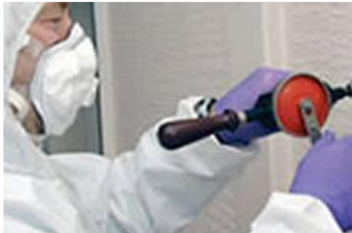
Asbestos textured coating on wall
