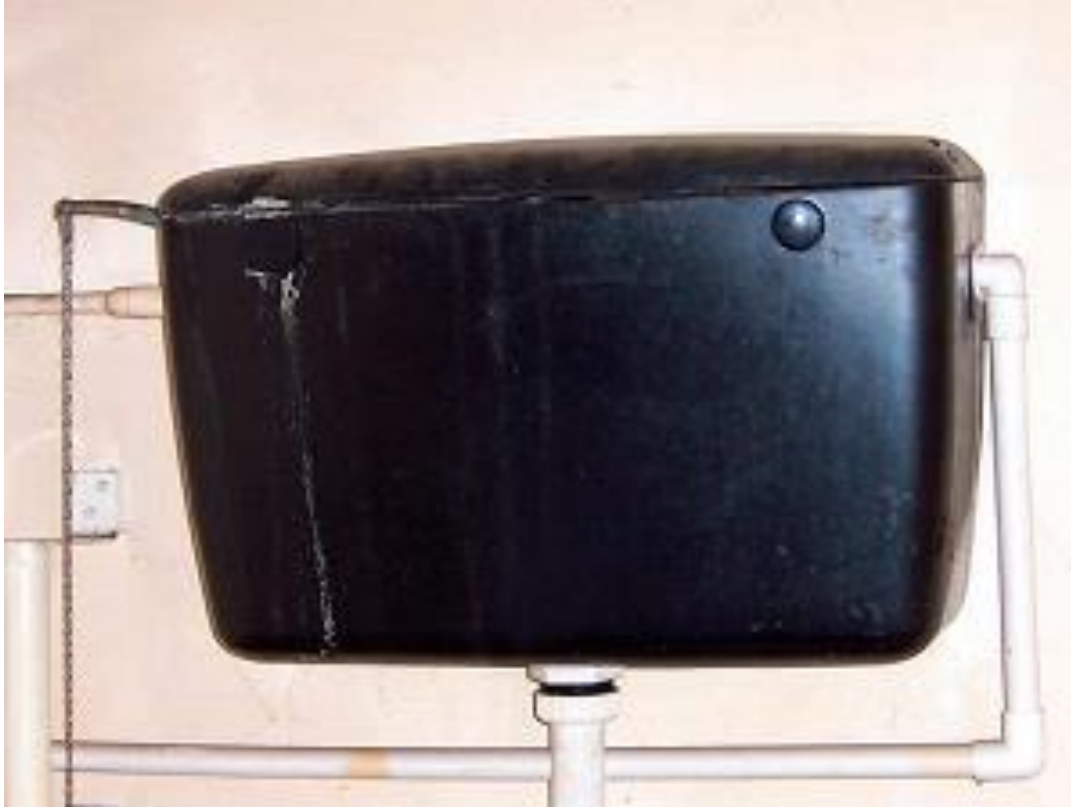
Toilet cistern containing asbestos reinforced materials
