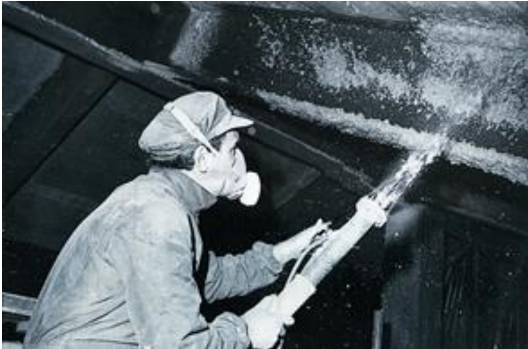
Under Roof Spray Coating
