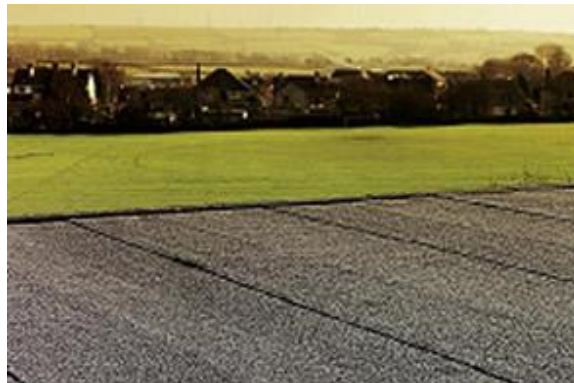
Asbestos roofing felt
