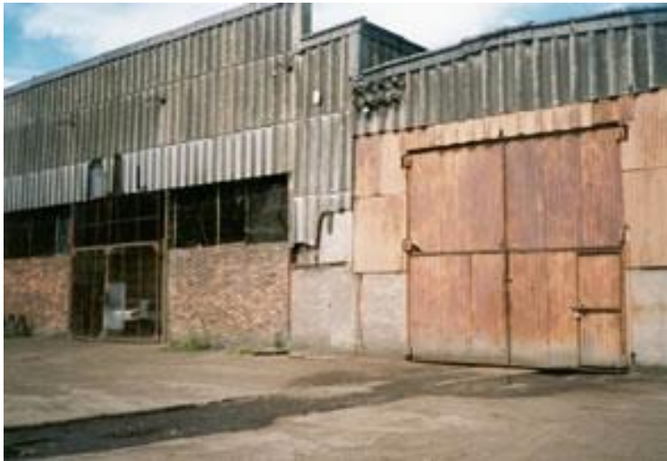
Asbestos cement wall cladding on warehouse
