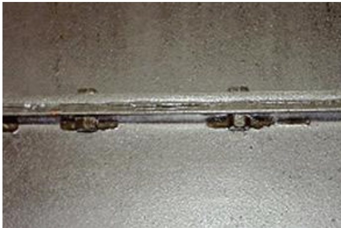
Asbestos string gasket between metal sheets
