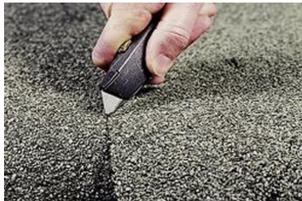
Asbestos roofing felt being cut
