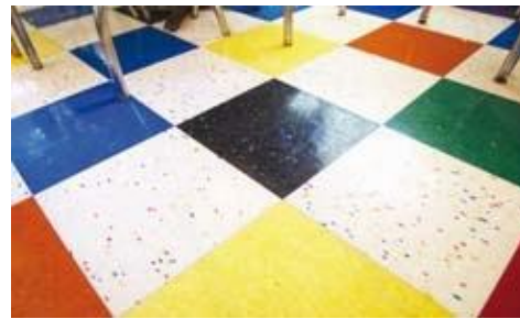
Asbestos-containing floor tiles
