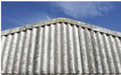
Asbestos cement wall cladding
