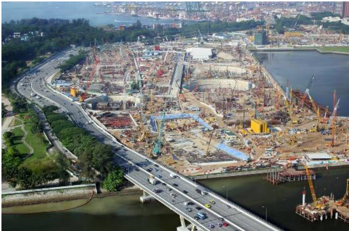
Mega construction site Marina South, Singapore
